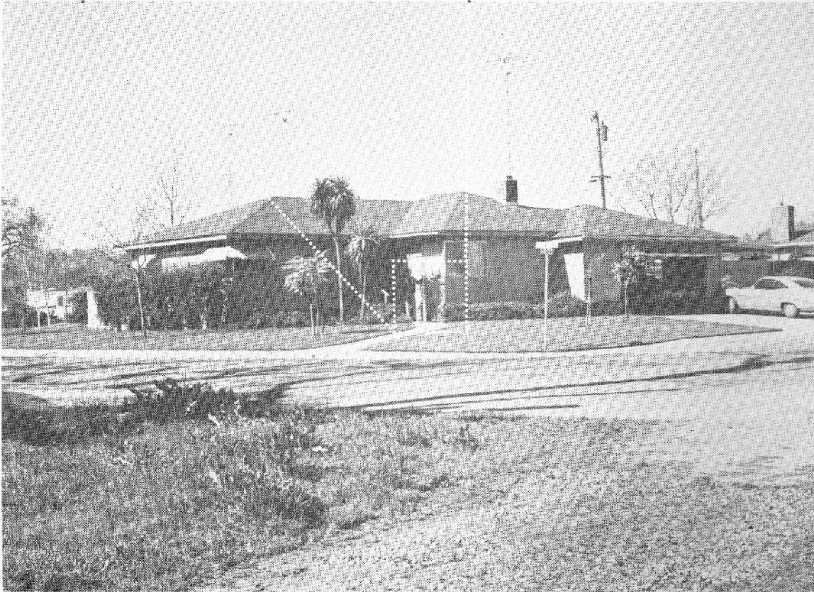
Figure 18 - Future flood heights, Cirby Creek at Tina Lane and Coloma Way.
