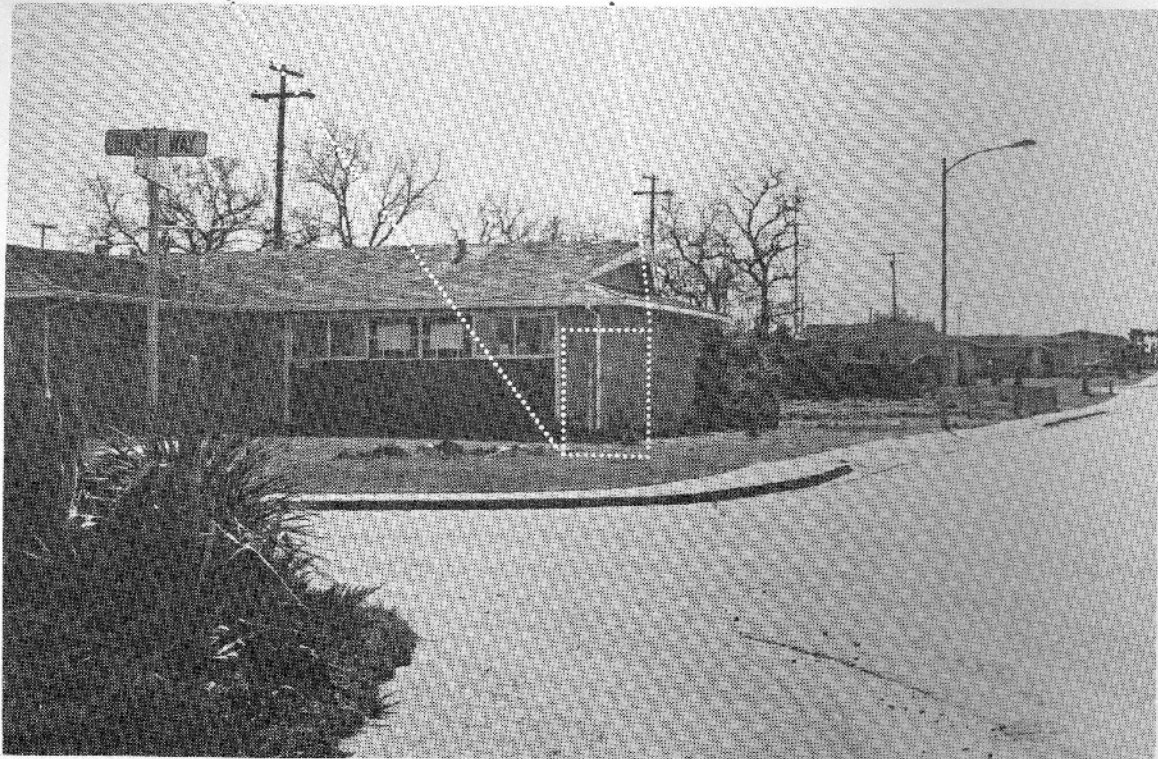
Figure 20 - Future flood heights, Linda Creek at Champion Oaks Drive and Hurst Way. See Figures 11 and 12, page 17 for flood conditions at this location.
