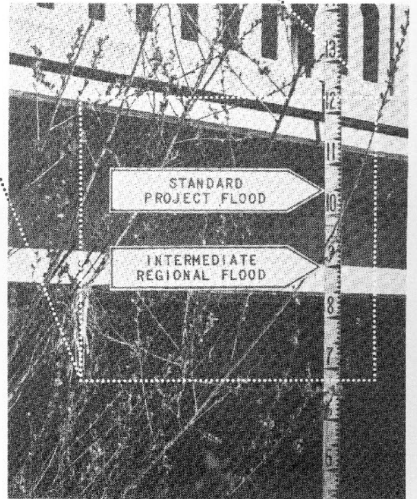
Figure 17 - Future flood heights, Antelope Creek at Atlantic Street (downstream side of bridge).
