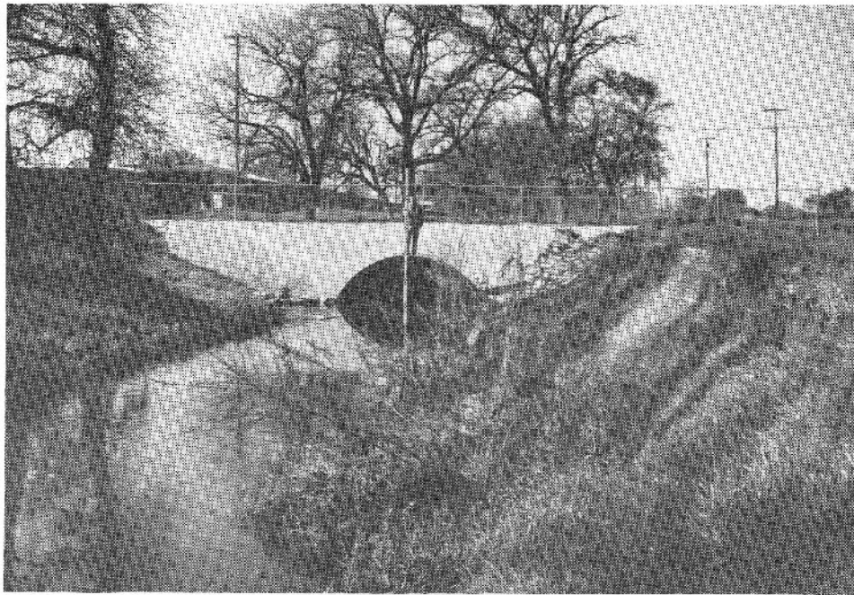
Figure 7 - Culvert on Linda Creek at Champion Oaks Drive.
